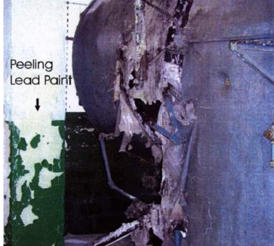
Figure 4 Building 203 (Heating Plant) Suspected Asbestos (April 2002)
