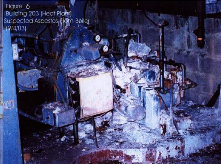
Figure 4 Building 203 (Heating Plant) Suspected Asbestos (April 2002)
