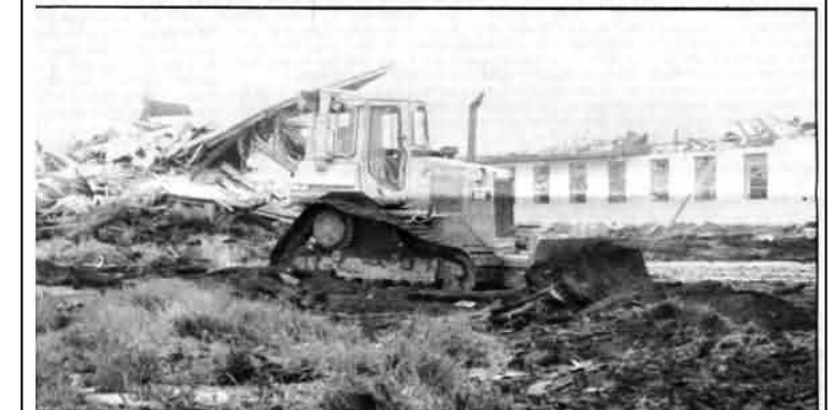
The demolition was complete. The burial was taking place. Deep holes were dug and the remains of the buildings pushed in and covered up. 6-9-93
