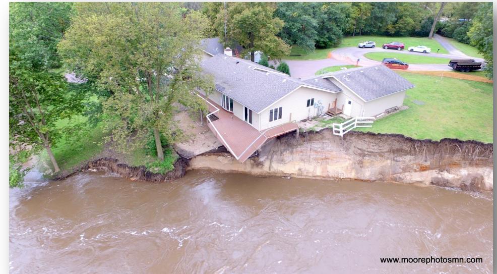
*House on the banks of the Le Sueur river, later demolished due to impacts of erosion
